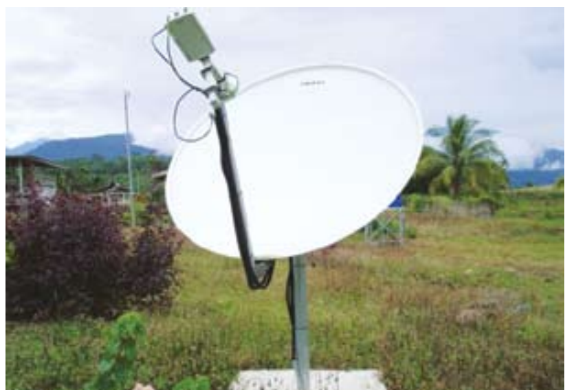
The satellite system at SK Tagop Darat Ranau
